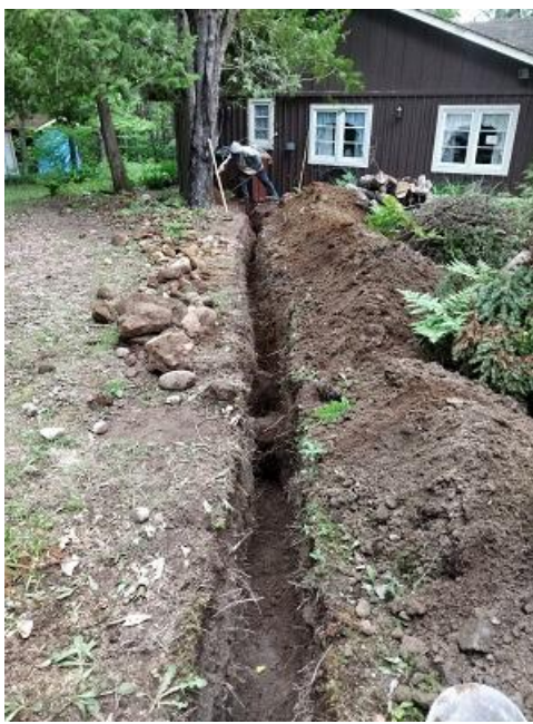
The long trench!
